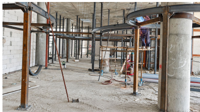
Steel framing / installation
