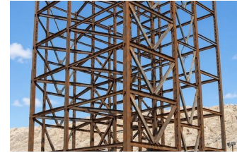
04 Structural Frame Assembly
