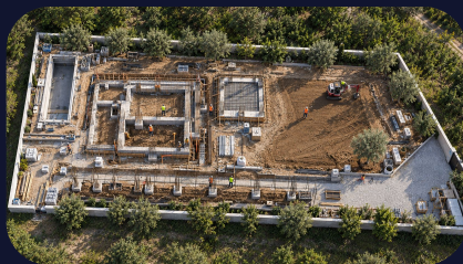
02 Foundation / Early-Works Study
