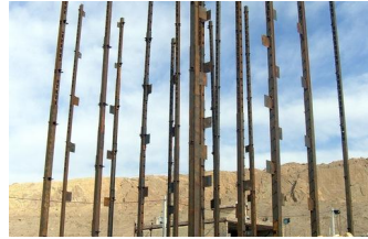
03 Steel Column Erection
