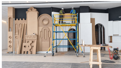
Frontage / finish installation
