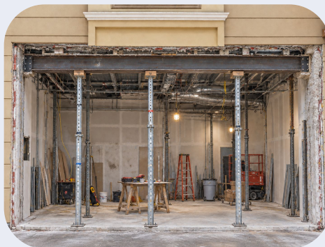
02 Opening & shopfront preparation
