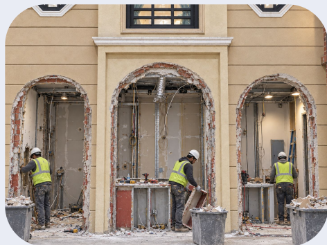
01 Existing condition & strip-out
