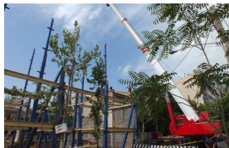
03 Steel Erection — Lifting Operation
