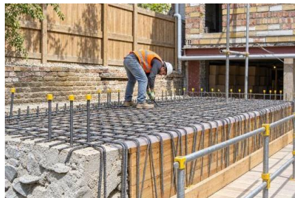
Foundation reinforcement / workmanship
