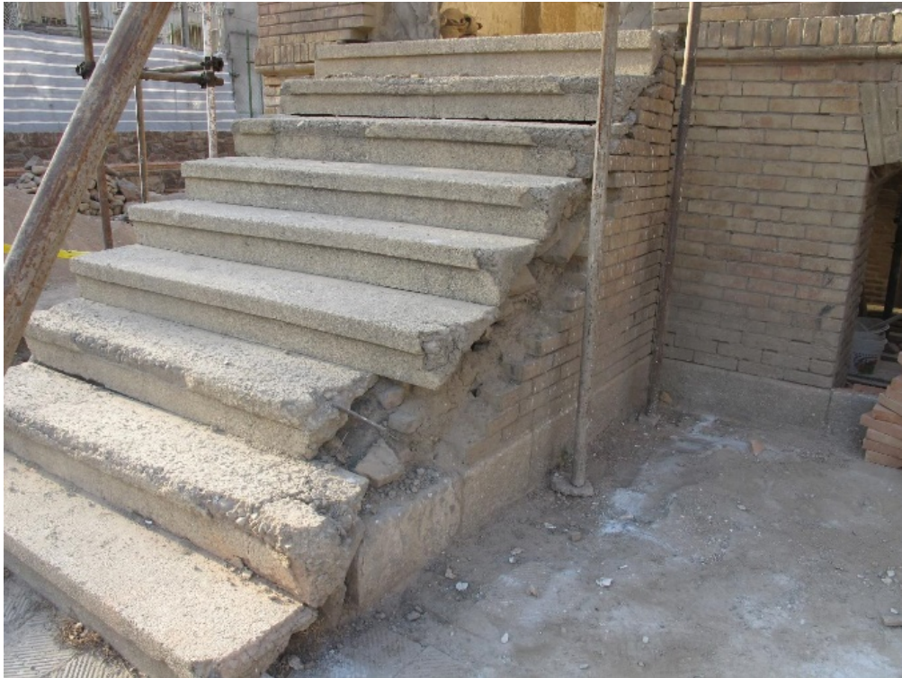
Image 11: The use of single-piece terrazzo as the final stair finish during the early second Pahlavi era.
