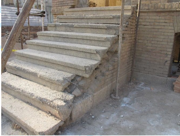
Image 1: The use of single-piece terrazzo as the final stair finish during the early second Pahlavi era.
