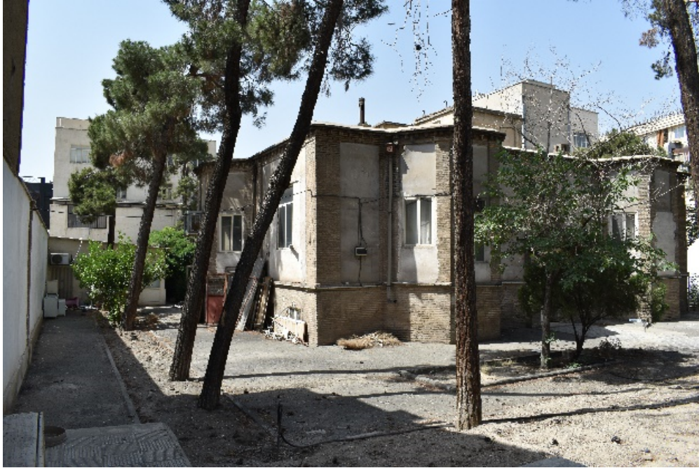
Image 6: The north façade of The Glass and Mirror Union Mansion
