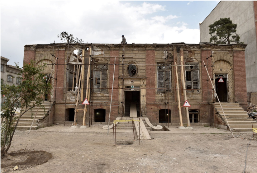
Plate 3. The south façade has sufficient evidence of an earlier state of the fabric that refers to the principle of restoration policy
