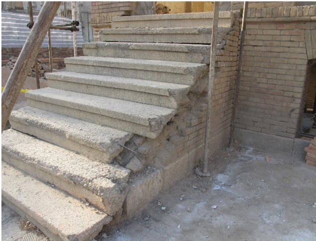
Plate 4. The use of single-piece terrazzo as the final stair finish during the early second Pahlavi era
